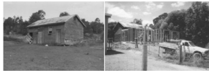
Blackwood Police stables before renovations in 1977 and 1998 with Allan Hall and Brian working on the Historical Society's Museum extensions at the back. Photos courtesy Margot Hitchcock.
